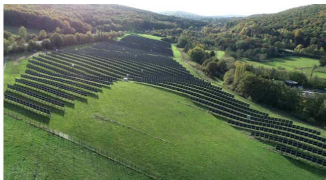
Fig. 51: Eppelborn-Dirmingen solar farm with 2 MW p with vertical solar fences by Next2Sun. © Next2Sun GmbH
