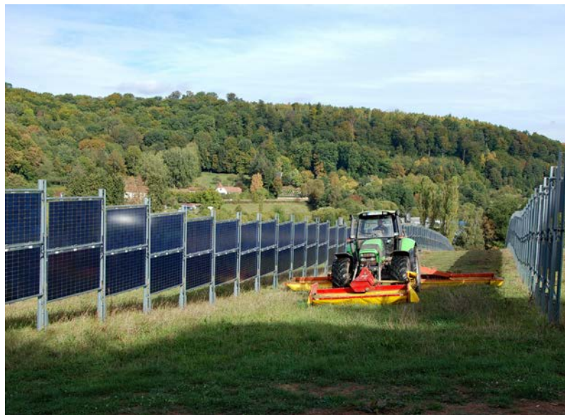
Fig. 31: Vertically deployed, bifacial PV modules used within the agrivoltaic system in Eppelborn-Dirmingen, with 2 MW p of capacity, built by Next2Sun. © Next2Sun GmbH
