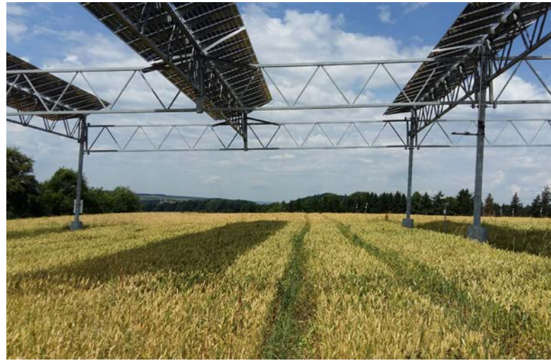
Fig. 48: The shaded strips underneath the PV modules move with the sun's position. © University of Hohenheim.
