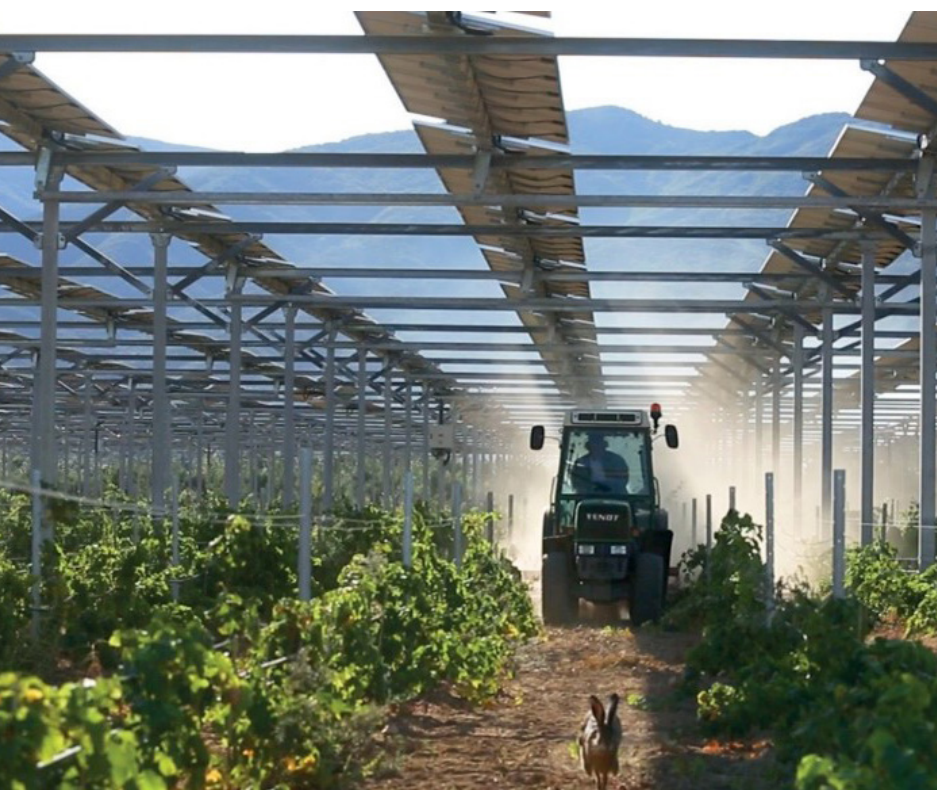
Fig. 44: Overhead system with continuous rows of PV modules.
