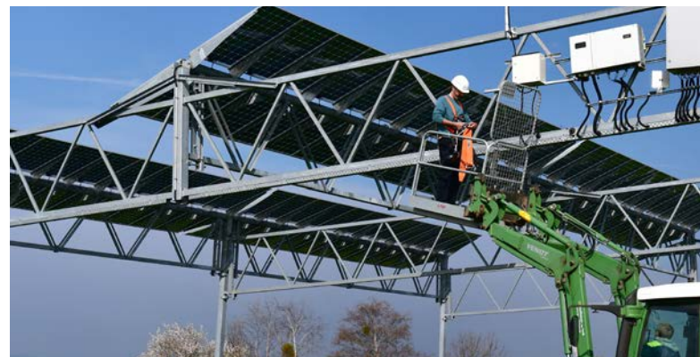
Fig. 54: Maintenance work on the agrivoltaic system in Heggelbach. © Fraunhofer ISE
