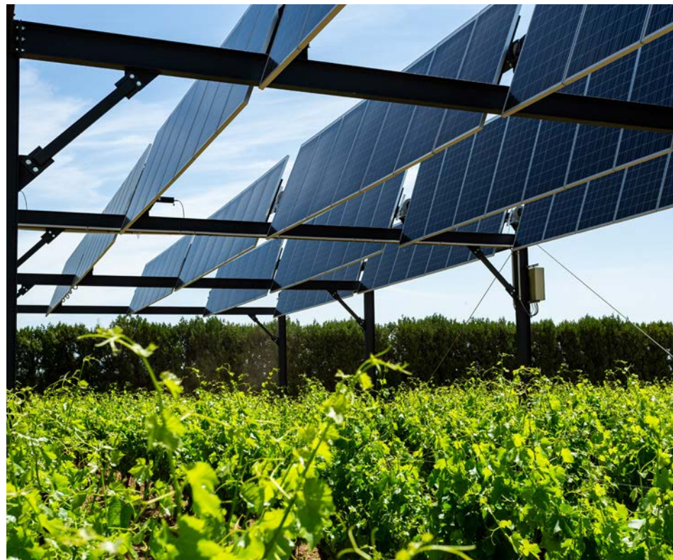
Fig. 45: Single-axis tracker system on a demonstration system in France. © Sun'Agri
